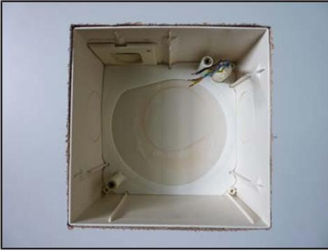
3. Place the seal, included in the scope of delivery, on the housing floor. When doing so, pay attention to the guide edges of the seal.
