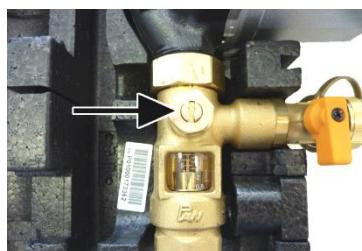
➤ Open the flow counter ball valve (→ arrow).
