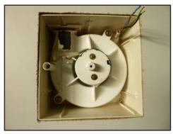
2. Remove the white seal on the housing floor.
