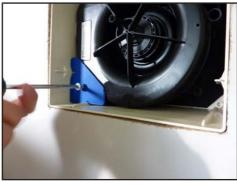
For ER-A: continue with step 3. For ER-AK, ER-AH, ER-AB, plug cover's flat cable with plug into interface connector. Ensure correct connection.
