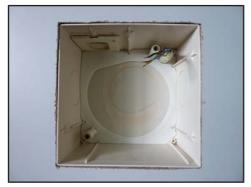
Place the seal, included in the scope of delivery, on the housing floor. When doing so, pay attention to the guide edges of the seal.
